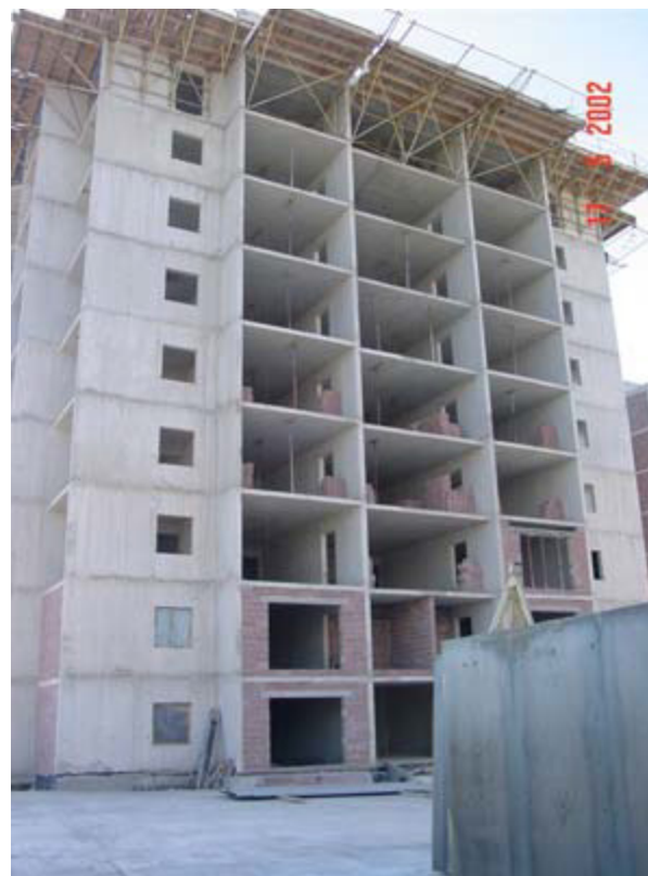
Figure 10: A Typical Tunnel Form Building Nearing Completion (Note Masonry Façade Elements)
